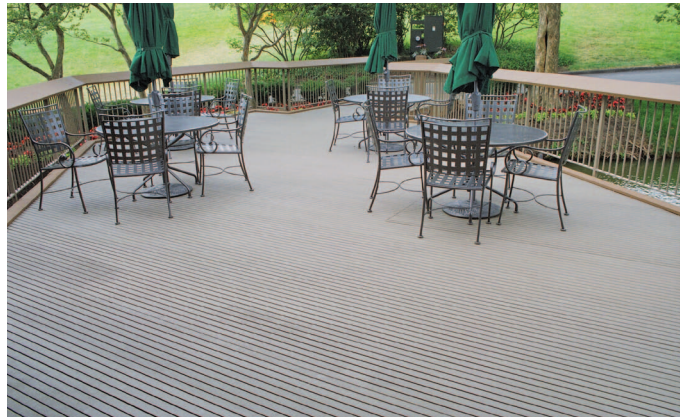
The Muirfield Village Golf Club, designed by Jack Nicklaus, offers an outside patio deck for players to relax and have a snack between nines. After years of constant moisture and the steady pounding of golf shoes, the wood deck had become a safety hazard and required replacement. Strongwell manufactured DURAGRID® T-1800 using a custom pigmented resin to replace the wooden deck to offer both the aesthetic and structural benefits the club was looking for.
