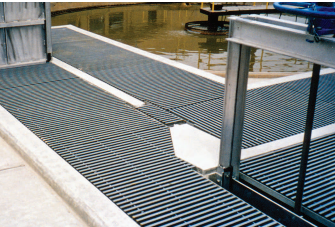
Low maintenance fiberglass grating provides trouble free operations for the covers and walkways in the Lakewood, Colorado Wastewater Treatment Plant Headworks. DURADEK® I-6000 1-1/2" was used.
