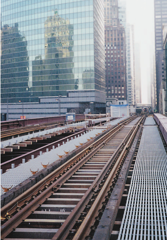
Chicago Transit maintenance walkways alongside elevated train tracks constitute one of the largest fiberglass grating installations in history. This project used DURAGRID® T-5000 2" with a custom polyester resin.
