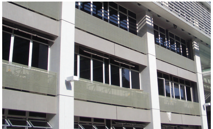
Strongwell DURADEK® I-6000 grating was installed at this School of Business and Information Systems in Hong Kong as air-conditioning platforms when placed horizontally and as louver when placed vertically (as shown here).
