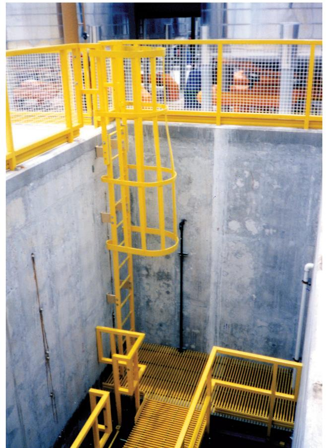
Fiberglass access ladders are used throughout the service areas of Sea World in Orlando, FL, and resist saltwater corrosion and reduce maintenance costs.
