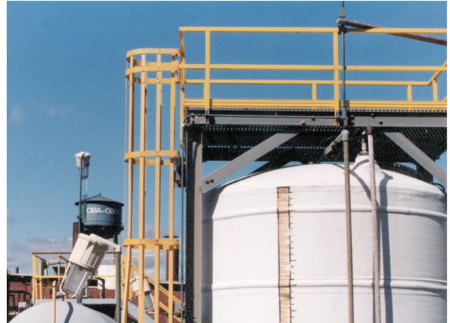
This fiberglass ladder and cage provide worker access to a maintenance platform at a Ciba Geigy plant in the northeastern United States.
